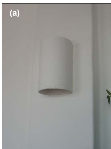
(a) Wall-mounted up/down lighting (b) Wall wash creates a glow visible from the nesting beach
