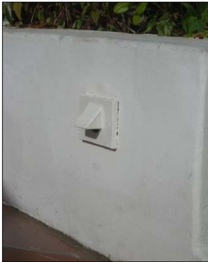
Wall-mounted stairway steplight with visor
