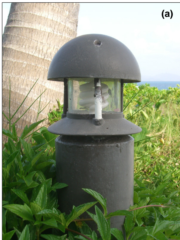
(a) Unshielded bollard (b) Light from the unshielded bollard reflects on villa walls, causing indirect light known as "wall wash"
