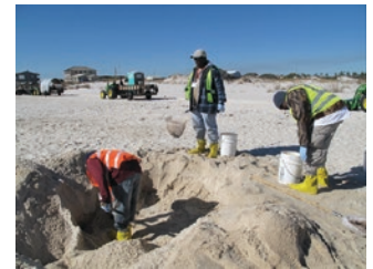
Figure 4.18. Manual removal of residual oil during the Deepwater Horizon spill in the Bon Secour National Wildlife Refuge, Alabama. Mechanical equipment was permitted for logistical support and to transport the manually recovered oil. Photo: NOAA.
